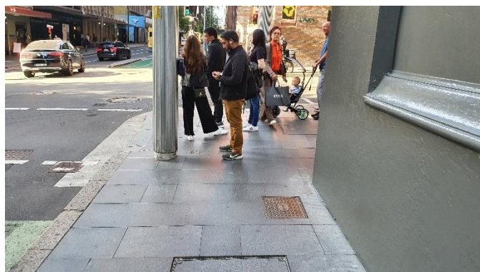
Figure 23: Kent / King St intersection – south-east corner, showing pinch point of the lamp/traffic signal pole.
